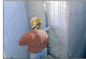
Mortar spraying on polystyrene panels with welded wire meshes
