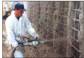
Spraying concrete
