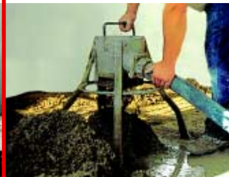
It pumps it quickly up to 40m in height
