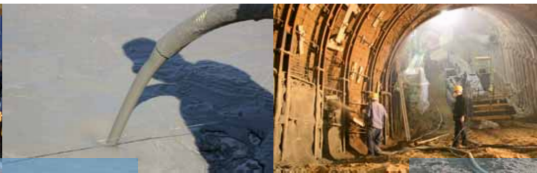
Foam concrete pumping
